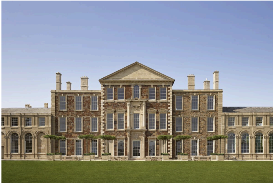
The 400-year-old, grand, imposing building is now RH England. Photographer: Courtesy of RH England
