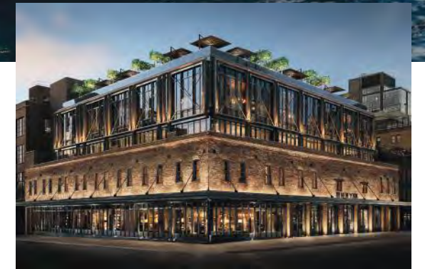
Above and below: the RH New York gallery showcases home furnishings over 90,000 square feet, plus a rooftop restaurant
