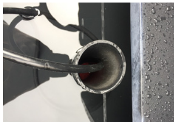
Image 3: Feed the plug/cord into the hole.
