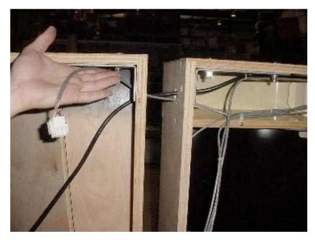
3. Feed the three pin and then two pin cables through the holes n the alley and the back cabinet and pull them through.
